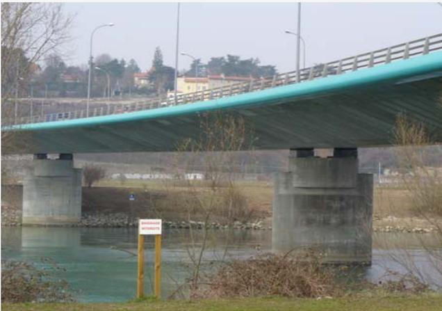
Resin-polymer vibration absorbers between span beams and columns (Bridge over the Rhone river, Villeurbanne, France)
