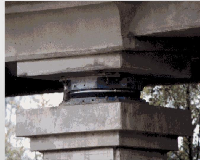
Friction Pendulum Bearing in the “American River Bridge”
