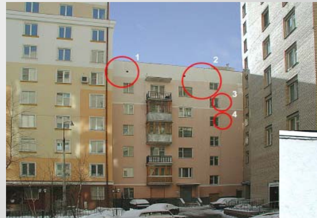
Cracks in an apartment house
