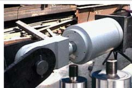
Forged dampers were used in the Torre Mayor Building. Developers-Paul Reichmann; architects-Ziedler Roberts Partnership (both of Canada)
