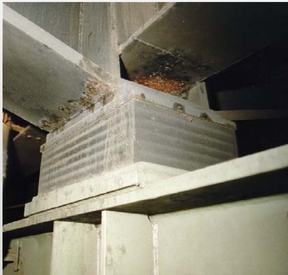
Laminated Neoprene mats for seismic protection by AARP (UAE)
