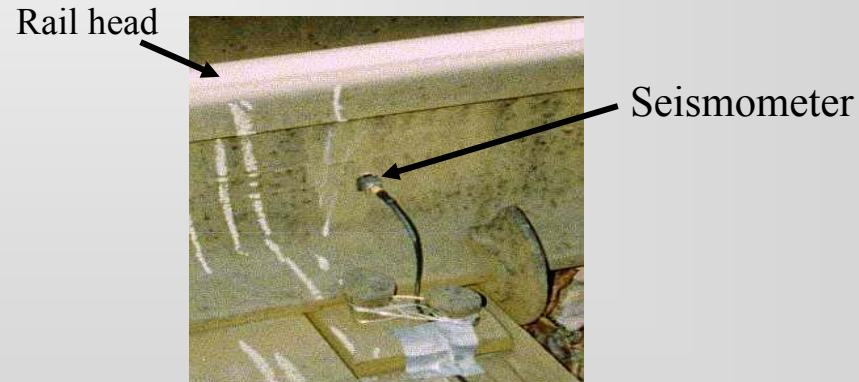
Crack determination in rails
